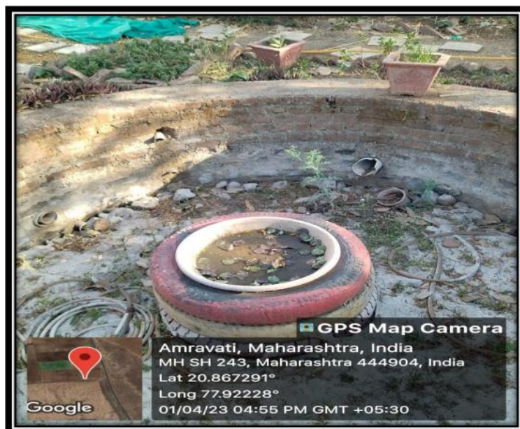
Rain Water Harvesting Pit
